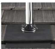
Acrylic coating helps prevent lead leaching. Can paint to match roof colour with acrylic house paint.
